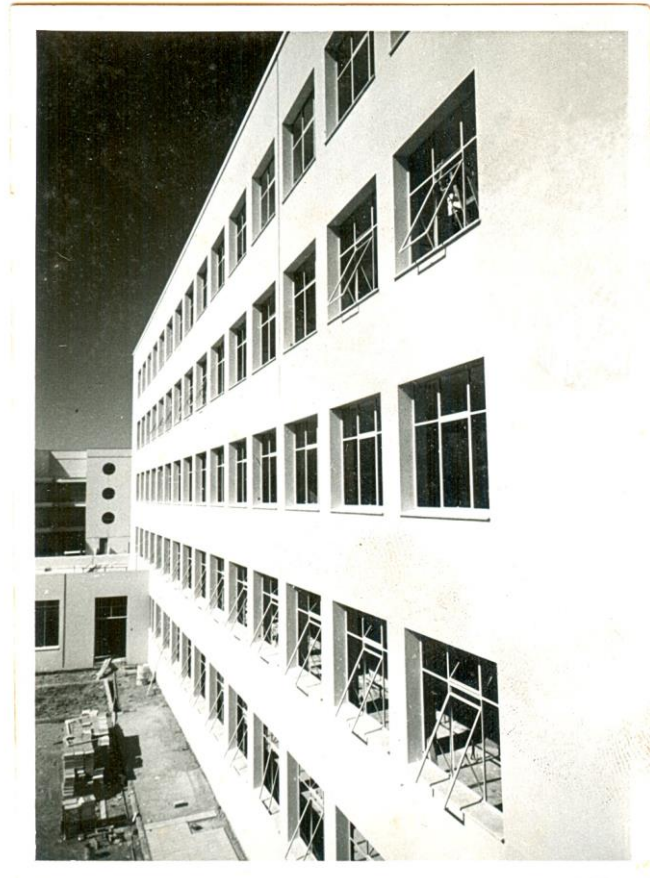
Figure 1: School of Dentistry under construction
